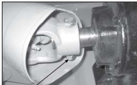
Figure 4-4 Shear Bolt Replacement
